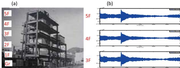
Fig.9 5-storey structure (a) and integrated displacements (b)
