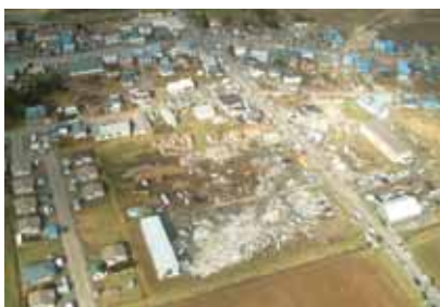
Photo 1 Overview of the damage (Photographed by F. Kobayashi)
