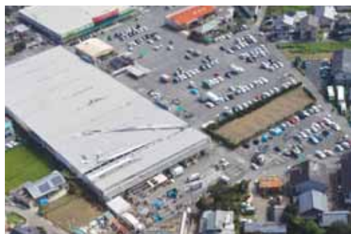
Figure 3 Damage to large-span building (Photo courtesy of Nobeoka City)
