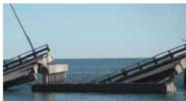
Photo 14: Damaged PC bridge in Biloxi
