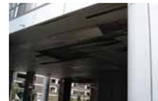
Photo 7: Damaged soffit
