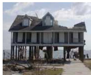
Photo 18: Damaged oceanfront elevated house
