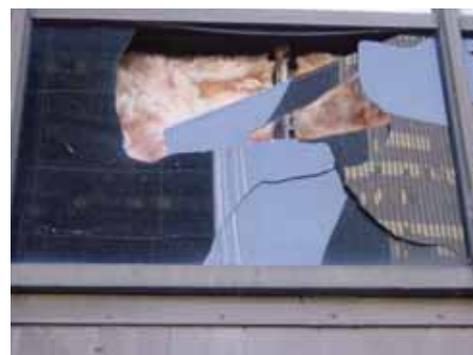
Figure 4: Broken window on North face of Hyatt Regency Hotel, likely caused by missile impact
