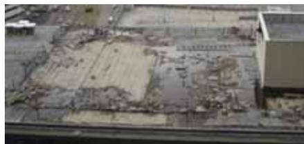
Photo 5: Slating on the roof of a building blown out by the wind
