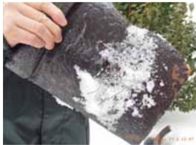
Photo 5: The damaged ridge tiles were conncted with metal wire
