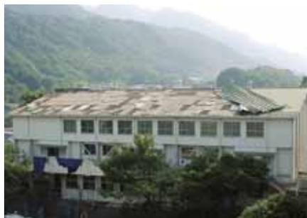
Photo 1: Damaged roof of gymnasium (T0511)
