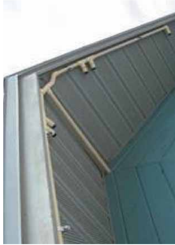
Figure 1. Photos of Wiring System and Roof Brackets for Instrumented House
