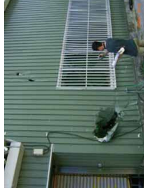
Photo 2. Damage to wall by a missile
