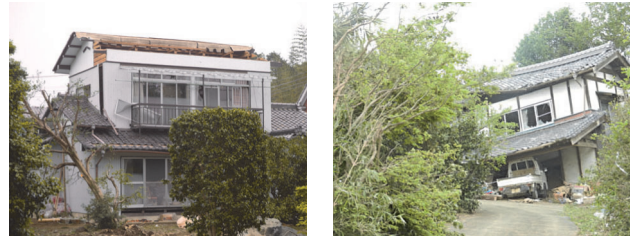
Fig. 4 Severely damaged structures
