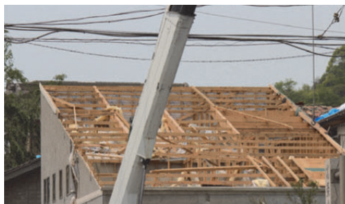
Fig. 12(f) Shed roof panel blown off
