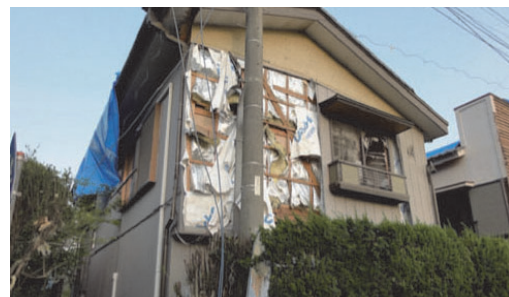
Fig. 12 (g) Damage to cladding
