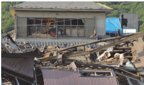
Fig. 12(d) and (e) Totally collapsed wooden houses in downtown area
