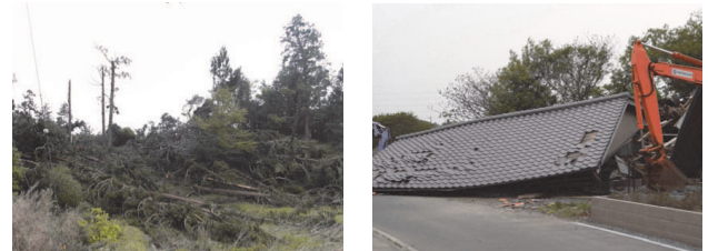
Fig.10 Fallen trees and totally collapsed storage
