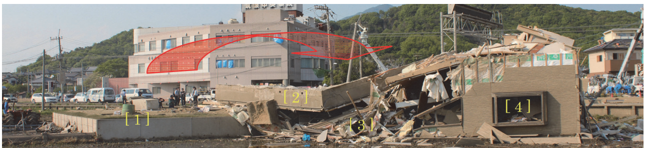
Fig. 12(a) Overturned house
