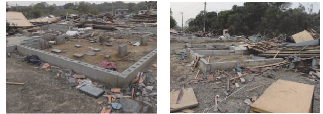
Fig. 9 7 houses totally collapsed
