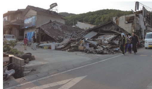
Fig. 12(d) and (e) Totally collapsed wooden houses in downtown area
