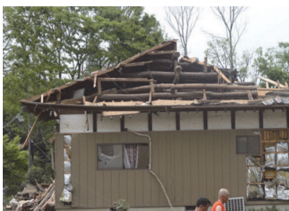
Fig. 12(f) Shed roof panel blown off
