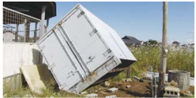
d. Storage tipping damage (area A)
