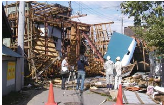
c. Wall and roof are partially overturned
