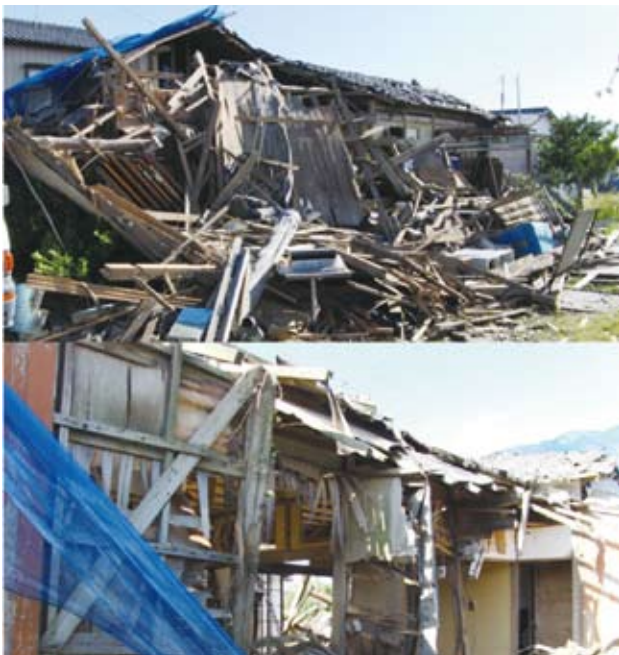
a. Half collapsed dwelling (area A)
