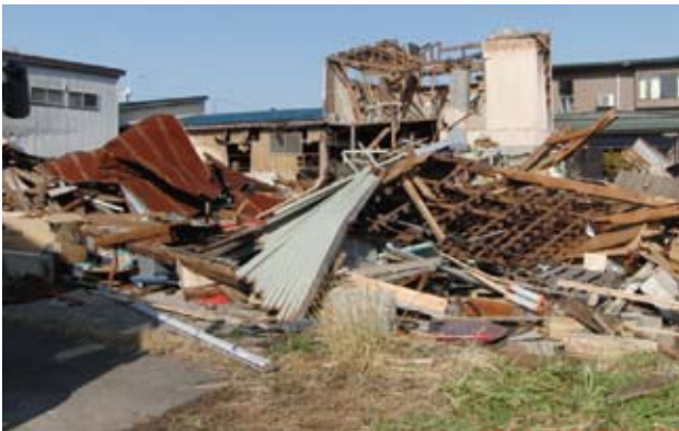
(point C) Fig. 23 Collapsed buildings
