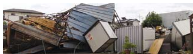
g. Complete-collapsed storage (point F) Fig. 4 Characteristic damage due to tornado
