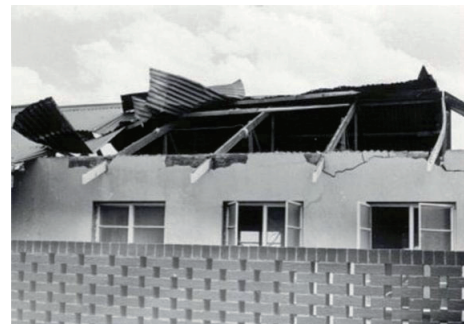
Figure 3b. Wind damage to a house
