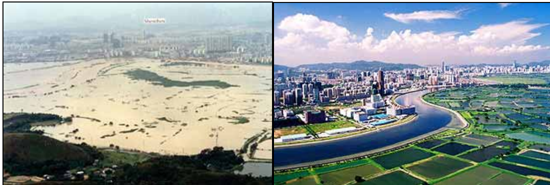
Figure 26: The Shenzhen River in 1993 (left) and in 2002, after flood control prevention (after Drainage Services Department, Government of HKSAR)
